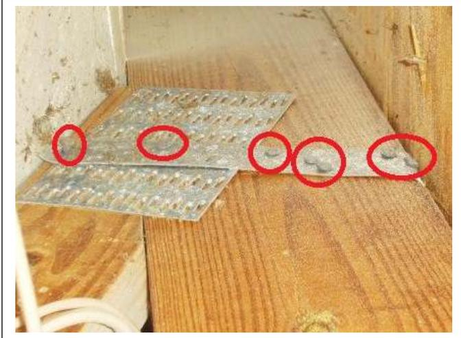
ROOF TO WALL ATTACHMENT – Properly installed
