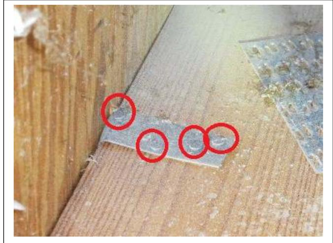
ROOF TO WALL ATTACHMENT – Properly installed
