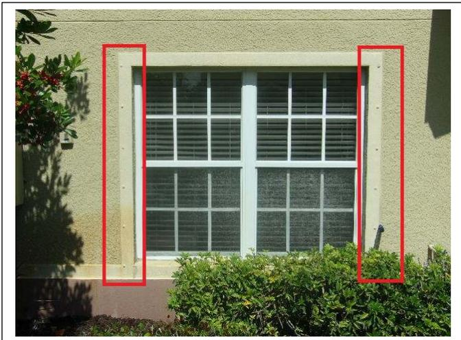
OPENING PROTECTION – Permanent shutter panel mounting hardware is properly installed at ALL window units.
