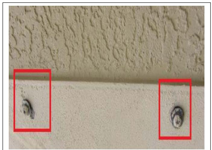
**OPENING PROTECTION** – Permanent shutter panel mounting hardware is properly installed at ALL sliding glass door units.
