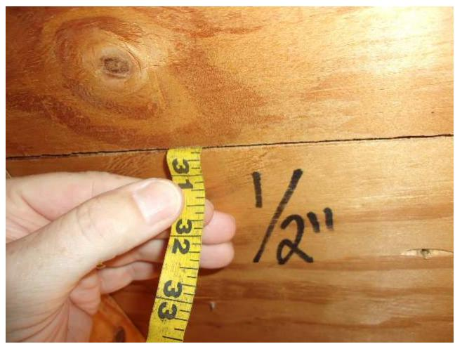
ROOF DECK THICKNESS –  $\frac{1}{2}$  inch plywood
