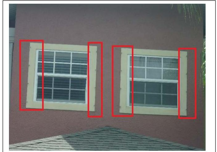
**OPENING PROTECTION** – Permanent shutter panel mounting hardware is properly installed at ALL window units.
