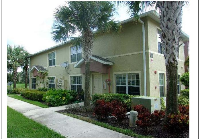
**OPENING PROTECTION** – The hinged entry doors cannot be identified as being impact rated, but local and FBC required the doors to be ASTM E-330 rated at a minimum.
