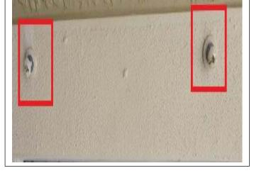
OPENING PROTECTION – Permanent shutter panel mounting hardware is properly installed at ALL sliding glass door units.
