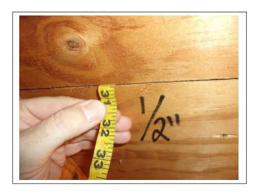
ROOF DECK THICKNESS –  $\frac{1}{2}$  inch plywood
