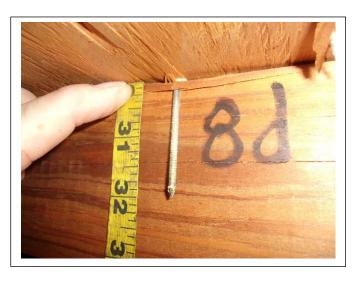
ROOF DECK ATTACHEMNT – 8d ring shank nails added in 2018. Roofing contract attached to this report.
