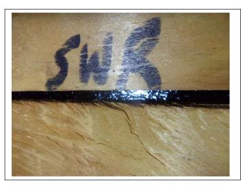
SECONDARY WATER BARRIER – A polymer adhesive (peel & stick) SWR Barrier was installed on the entire roof deck in 2018. Documentation attached to this report.
