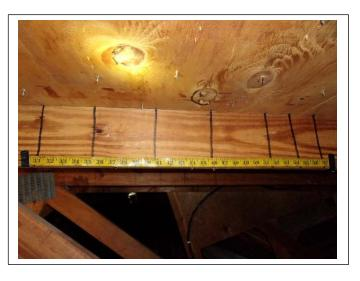
ROOF DECK ATTACHMENT – 8d nails within 6 inches in the field
