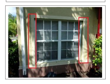
OPENING PROTECTION – Permanent shutter panel mounting hardware is properly installed at ALL window units.
