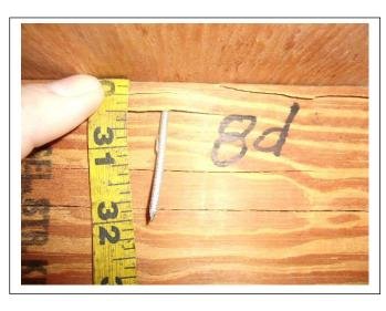
ROOF DECK ATTACHEMNT – 8d ring shank nails added in 2018. Roofing contract attached to this report.
