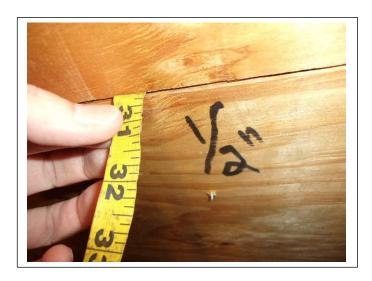
ROOF DECK THICKNESS - ½ inch plywood
