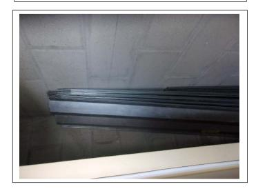
OPENING PROTECTION – Per local code and the FBC, large missile rated metal corrugated shutter panels are available to protect all glazed openings.
