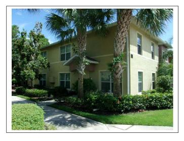
SIDE ELEVATION VIEW – The side entryway gables are not structurally connected to the main roofing system.
