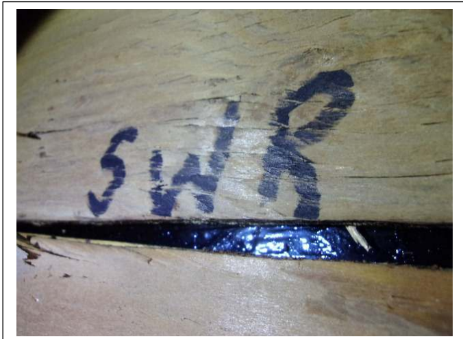
SECONDARY WATER BARRIER – A polymer adhesive (peel & stick) SWR Barrier was installed on the entire roof deck in 2018. Documentation attached to this report. NOA#15-0707.09
