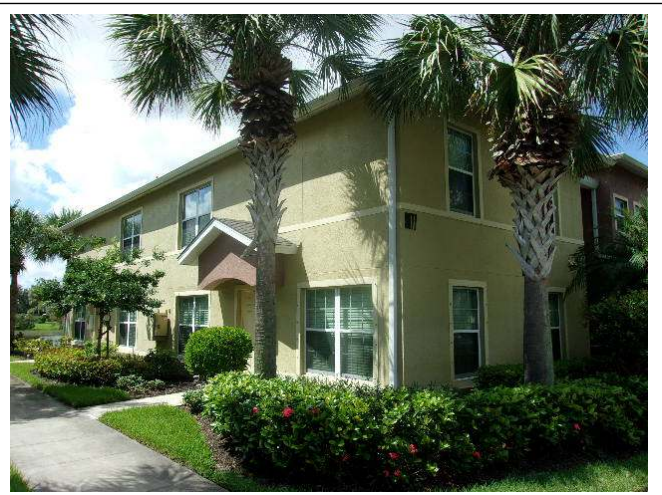
SIDE ELEVATION VIEW – The side entryway gables are not structurally connected to the main roofing system. They are attached to the reinforced walls.
