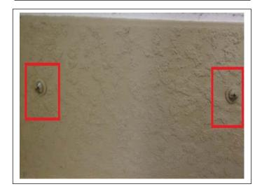
OPENING PROTECTION – Permanent shutter panel mounting hardware is properly installed at ALL sliding glass door units.
