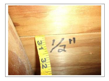
ROOF DECK THICKNESS –  $\frac{1}{2}$  inch plywood
