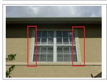
OPENING PROTECTION – Permanent shutter panel mounting hardware is properly installed at ALL window units. FBC# FL11964.1
