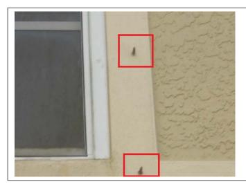
OPENING PROTECTION – Permanent shutter panel mounting hardware is properly installed at ALL window units. FBC# FL11964.1
