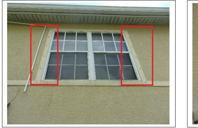
OPENING PROTECTION – Permanent shutter panel mounting hardware is properly installed at ALL window units. FBC# FL11964.1
