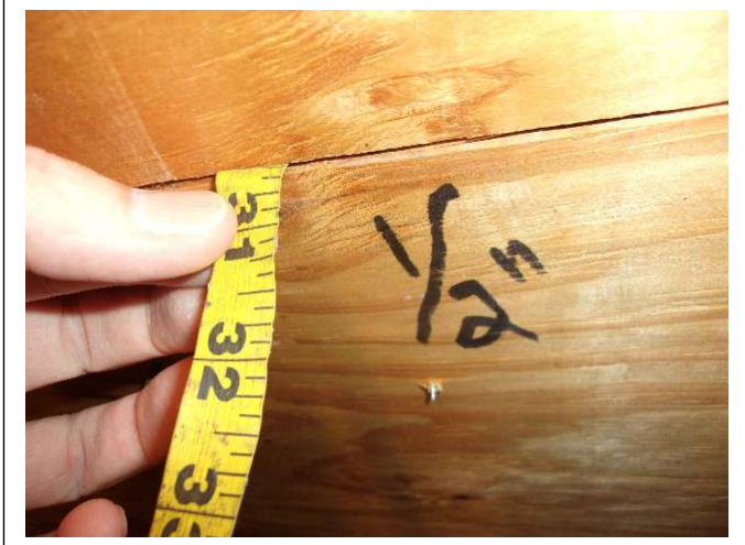
ROOF DECK THICKNESS – ½ inch plywood
