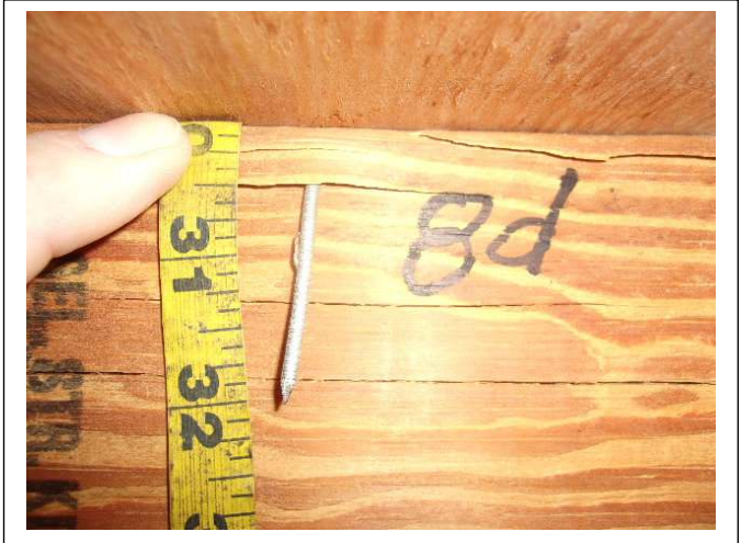
ROOF DECK ATTACHEMNT – 8d ring shank nails added in 2018. Roofing contract attached to this report.
