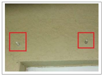
OPENING PROTECTION – Permanent shutter panel mounting hardware is properly installed at ALL sliding glass door units. FBC# FL11964.1
