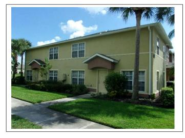
OPENING PROTECTION – The hinged entry doors cannot be identified as being impact rated, but local and FBC required the doors to be ASTM E-330 rated at a minimum.
