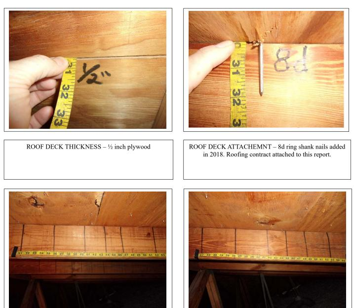
ROOF DECK ATTACHMENT – 8d nails within 6 inches along the edge
