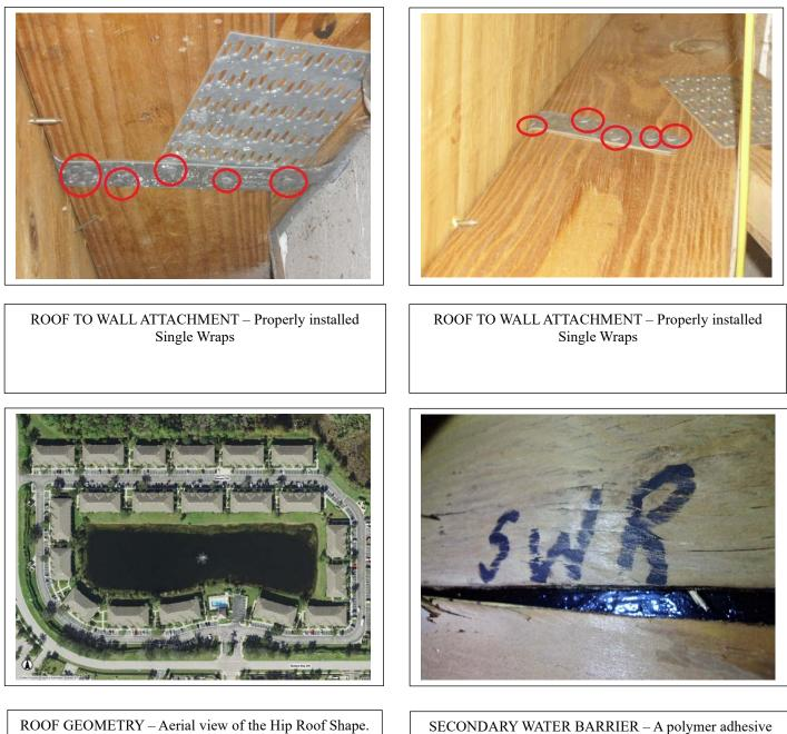
SECONDARY WATER BARRIER – A polymer adhesive (peel & stick) SWR Barrier was installed on the entire roof deck in 2018. Documentation attached to this report. NOA#15-0707.09
