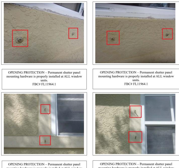
OPENING PROTECTION – Permanent shutter panel mounting hardware is properly installed at ALL window units. FBC# FL11964.1 OPENING PROTECTION – Permanent shutter panel mounting hardware is properly installed at ALL window units. FBC# FL11964.1
